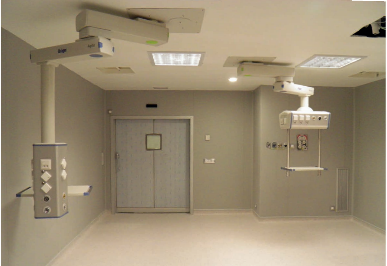
Hospital in Madrid, Spain
